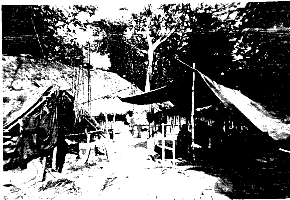
PIC: 3-A. B FULLY DESTROYED HOUSE.
