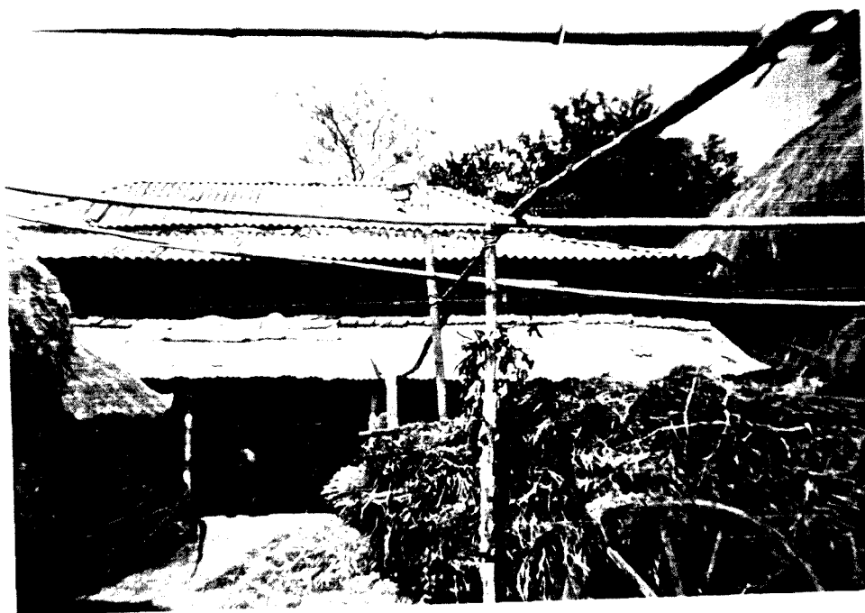
PIC: 3-B. PARTIALLY DESTROYED HOUSE.
