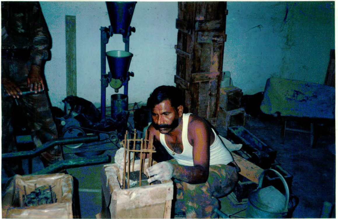
Photograph showing columns being jacketed by jacketing concrete and additional reinforcement.
