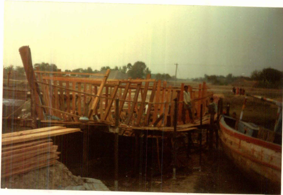
Fig.1: A bigger vessel being built in skeleton sequence in which the frames give the shape of a hull. In contrast, the traditional and small boats are built in shell sequence in which the planks give the shape of a boat.
