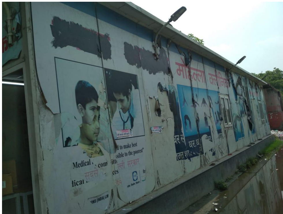
Figure 5.2: Water accumulated around the clinic. Photograph by author during field visit, July 2019.
