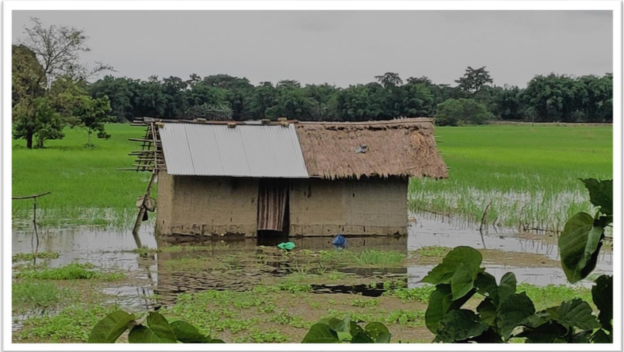
Photo 1: House inundated with flood. Source: The Author
