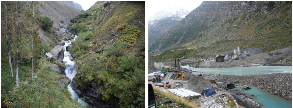
Plate 39: Sissu Nalah draining down from Sissu Slacial Lake (a) Construction activities at the periphery of Sissu town (b)
