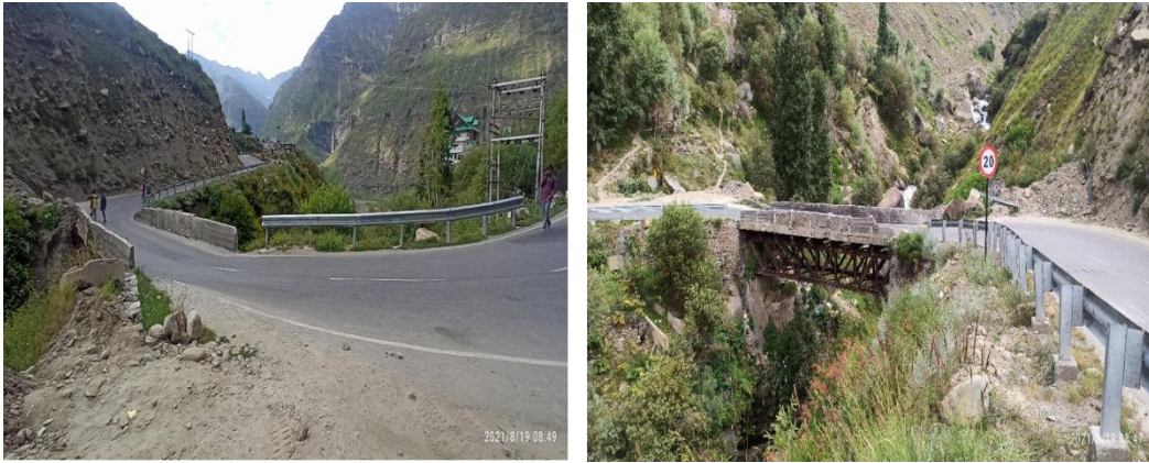
Plate 29: Field photographs of Leh-Manali Highway and Sissu Bridge impacted under Flood Inundated area.
