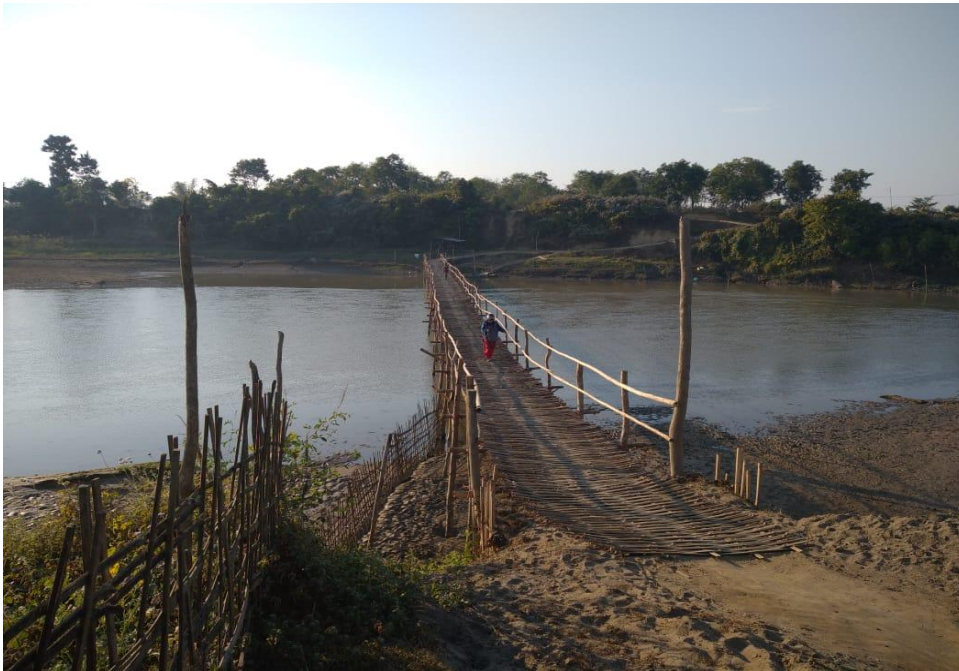
The narrow bamboo bridge on the river Doyang, which is a shortcut to Tengani
