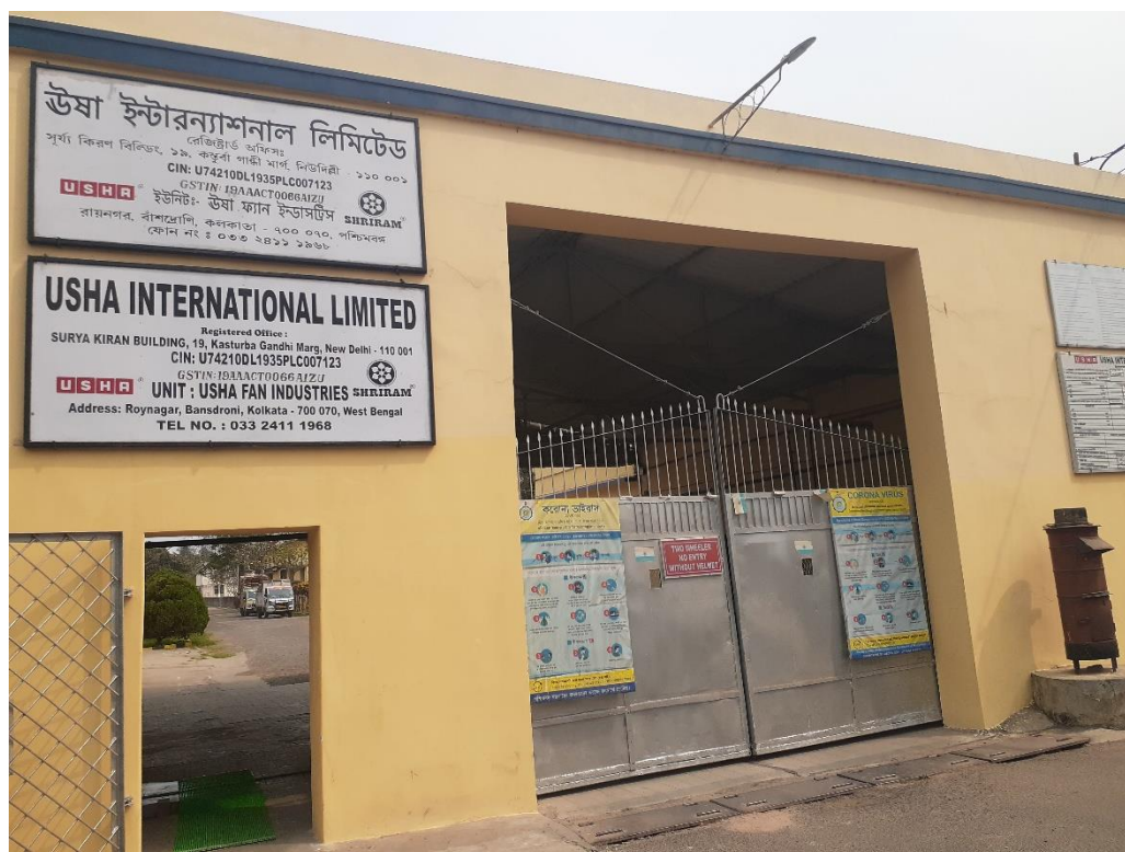
Figure 5.5. Usha Fan Division at Roynagar, Bansdroni, currently under Usha International Limited. Photograph taken during field survey in March 2021.
