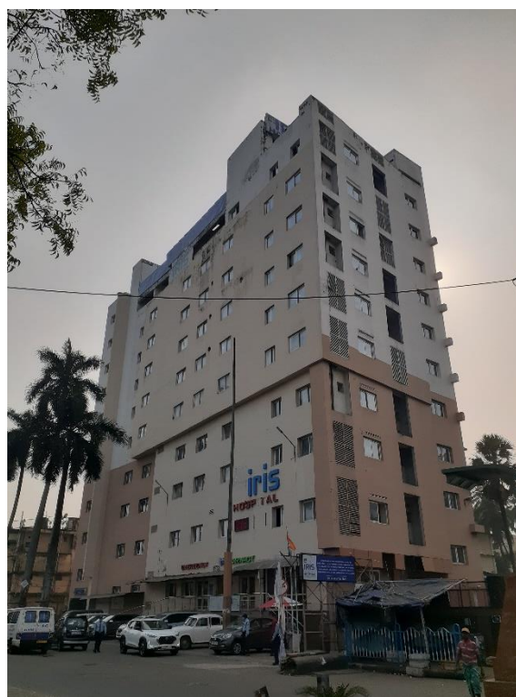
Figure 6.8. Iris Multispeciality Hospital, in Kusum Kanan (Dabur Warehouse) Photograph taken during field survey in September 2021.
