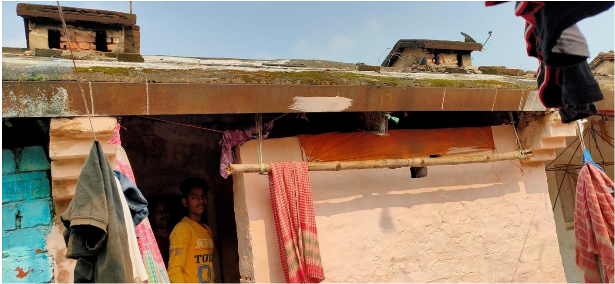
Figure 8: Showing Overall Housing condition of Reliance Jute Mill Quarter
