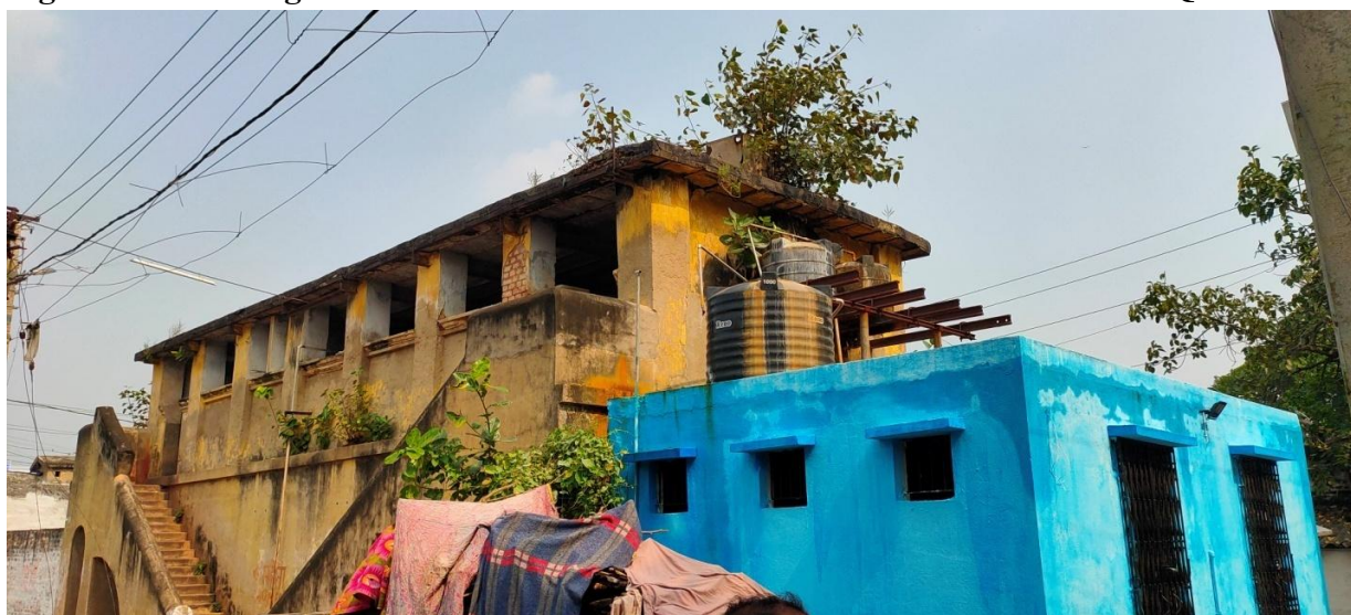
Figure 11: Showing Bathroom and Sanitation Facilities of Reliance Jute Mill Quarter
