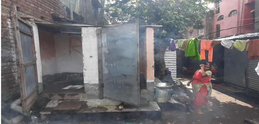
Figure 20: Public latrine facility in bastee line area in bastee line area
