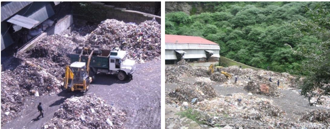
FIG. 3.9 A & 3.9 B - MUNICIPAL SOLID WASTE DISPOSAL PLANT AT DARNI-KA-BAGICHA Source: Photograph clicked by Researcher at the site during the field work
