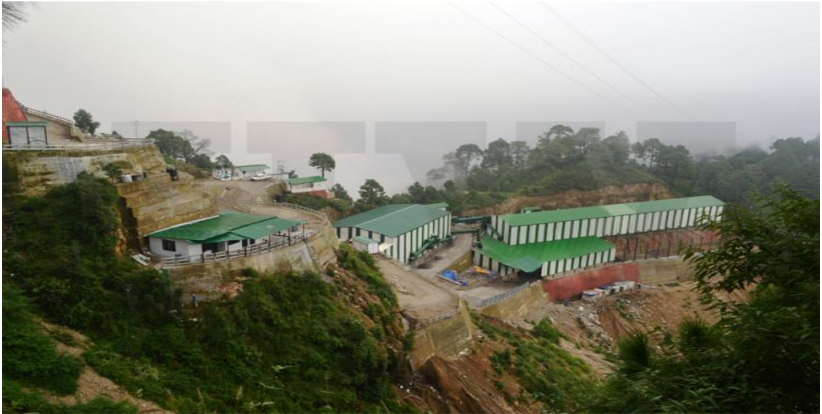
Figure: 3.12 New Municipal Solid Waste Treatment Plant at Bharyal on Totu-Tara Devi Bypass
