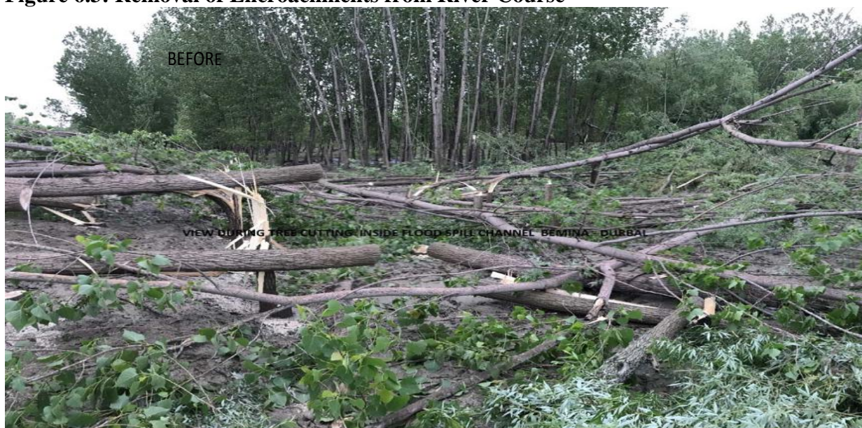
Figure 6.3: Removal of Encroachments from River Course
