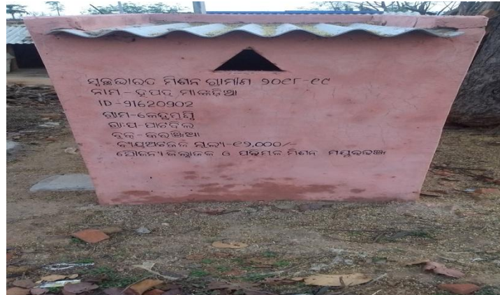
Figure 3.5: Newly Constructed Toilet in Study Village
