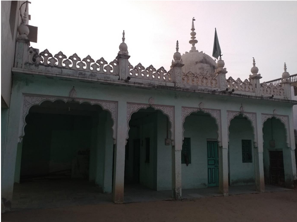
Figure 4.2: Dar-i Daulat Khan Masjid complex in Fatehpur.
