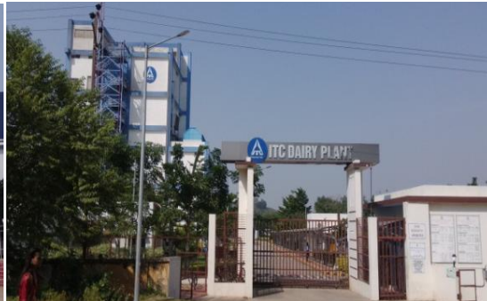
ITC Dairy Plant
