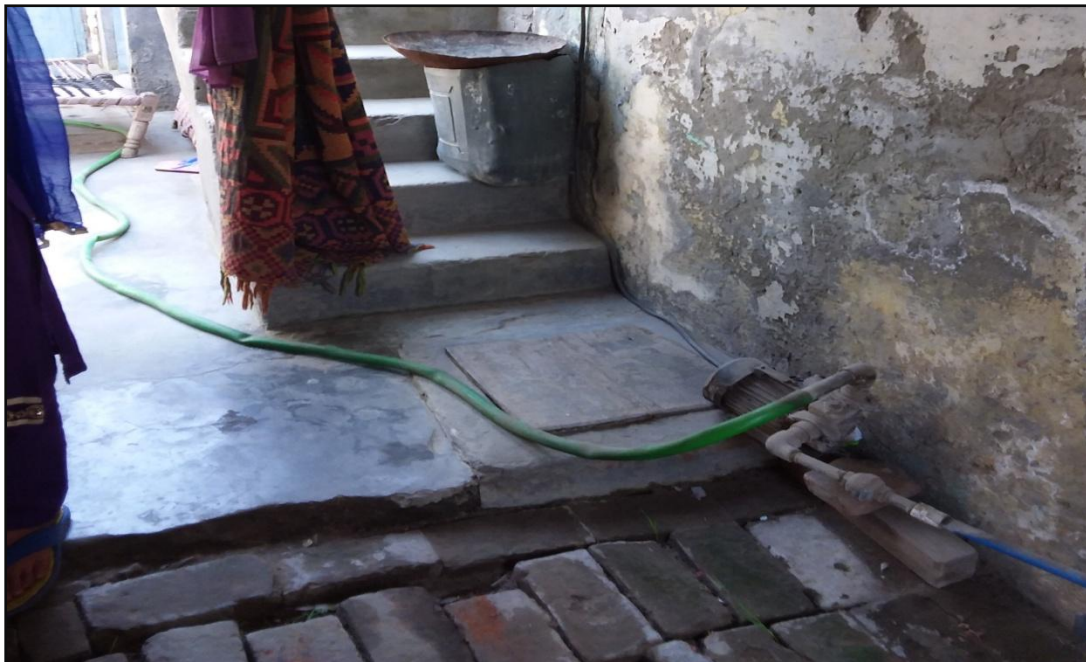
Pic.2 Use of the booster ( tullu pump ) to lift the water supplied by ULBs in Ajnala town, as the water pressure is low.
