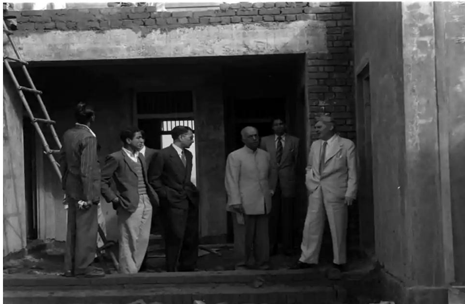
Image 9: Central Rehabilitation Advisor Mehar Chand Khanna showing an under-construction refugee quarter at Lajpat Nagar to British politician Aneurin Bevan on February 13, 1953.
