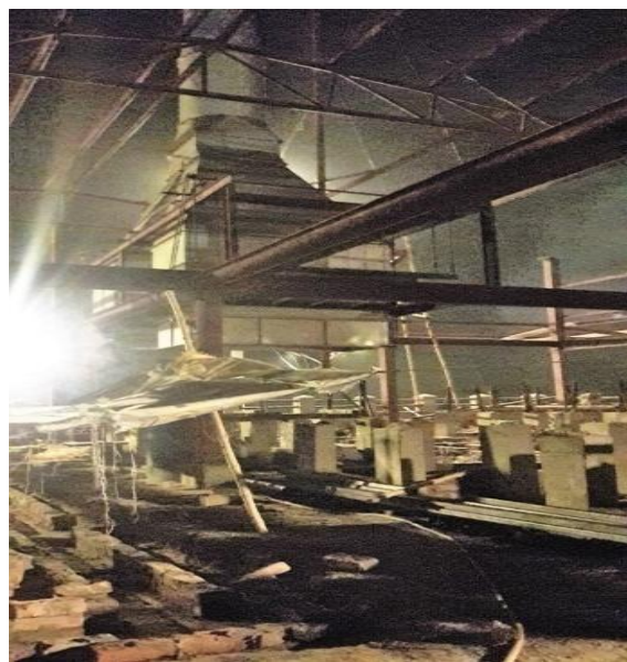
Funnel pipe connecting two cemented structure
