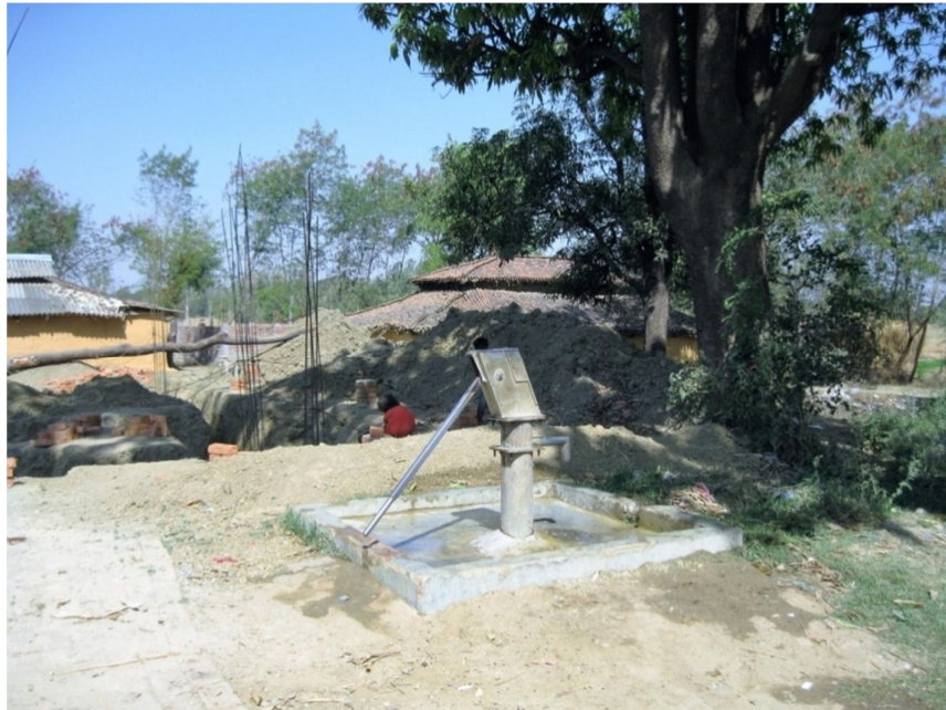
Photo 5: Hand pump near Power House, Kushmha
