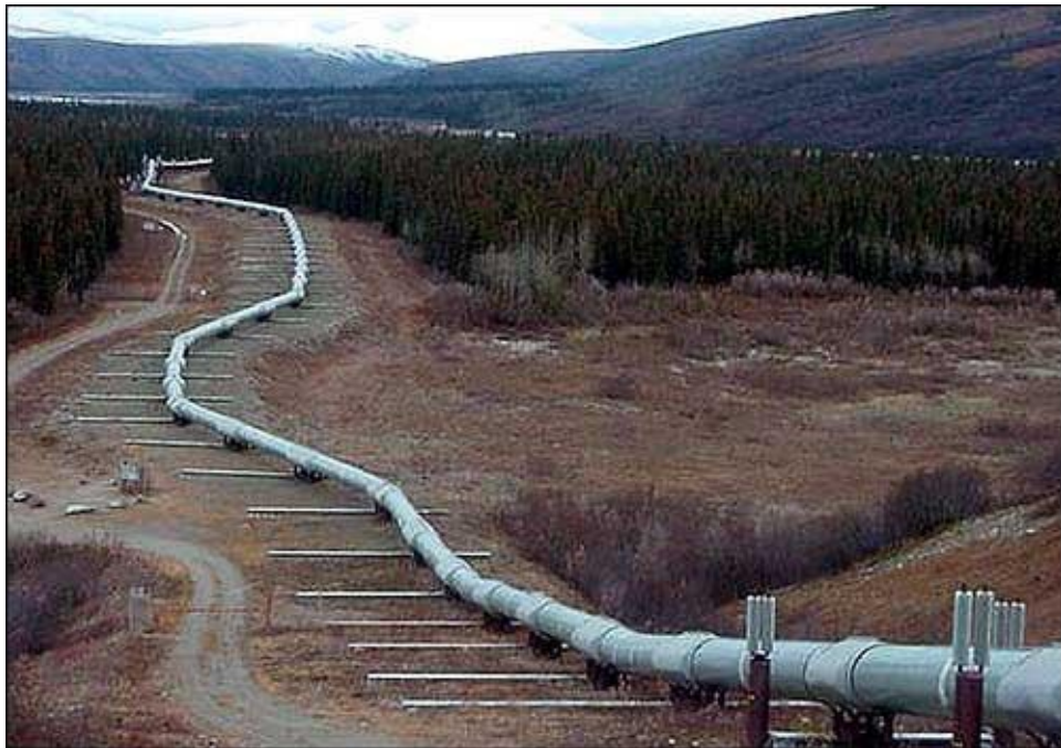
Figure1: Trans-Alaska oil pipeline
