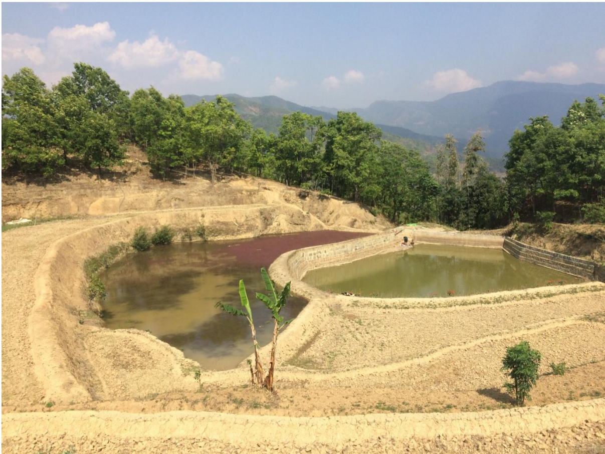
Figure B.1: Traditional Ruza (Rain-water harvesting ponds) in Kikrumba village
