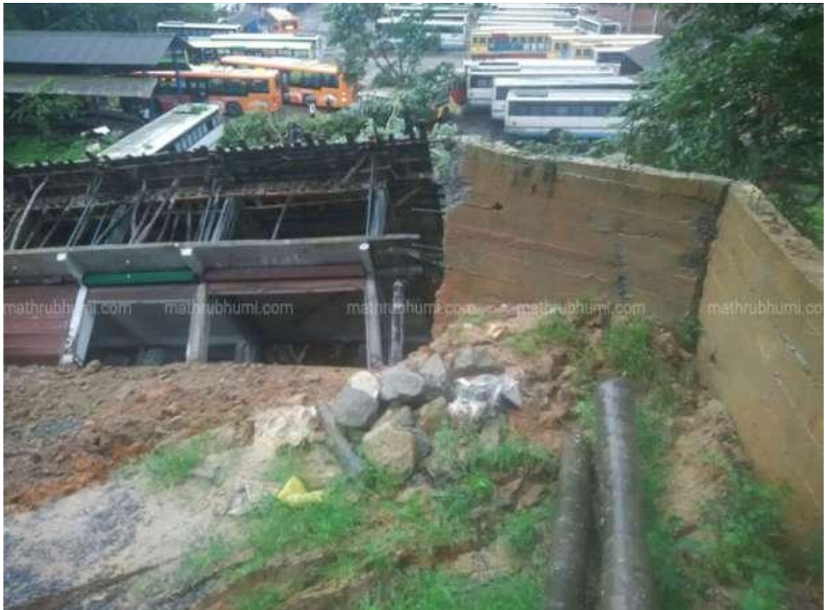
Picture 9. Collapsed building in Kalpetta
