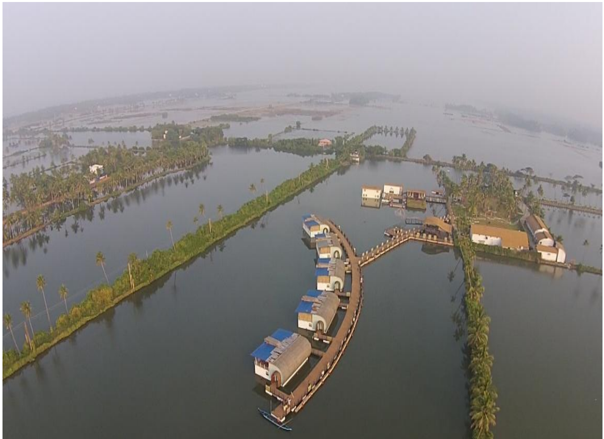
Picture 10. Sight of Aquatic Floating Resort constructed in backwaters
