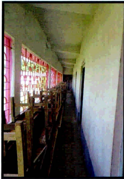
Figure 4: Benches are taken out of the rooms
