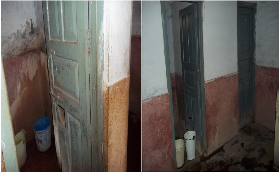
Picture 3.25 and 26: General Female Ward's Bathroom of Bareilly Mental Hospital
