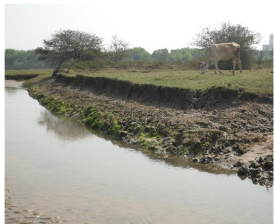
Figure 4.30 Eroded tidal creeks at Mahanadi confluence.
