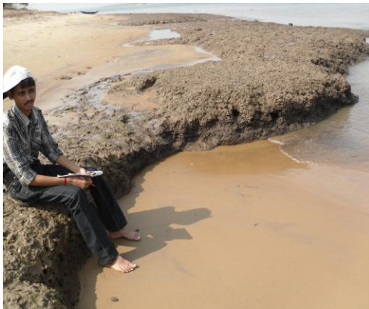
Figure 4.29 A part of projected headland exposed to erosion at Mahanadi confluence.
