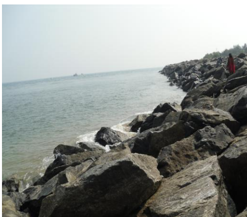
Figure 4.39 Sea wall protecting eastern side of projected head land. Sea wall construction results in near constant situation of shoreline after 1990's, which also responsible for insignificant net shoreline movement along transect 4, 5, 6 and 7.
