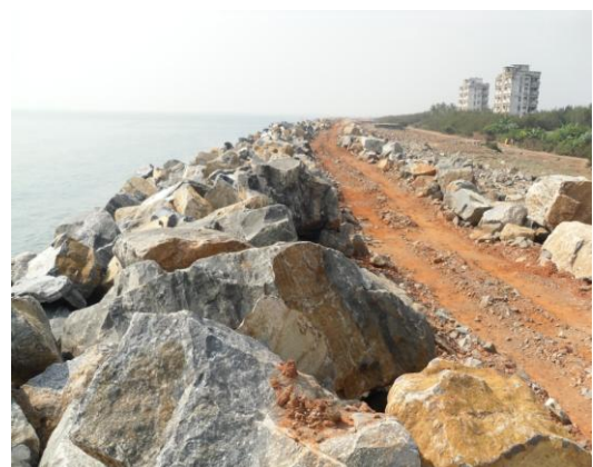
Figure 4.39 Sea wall protecting eastern side of projected head land. Sea wall construction results in near constant situation of shoreline after 1990's, which also responsible for insignificant net shoreline movement along transect 4, 5, 6 and 7.
