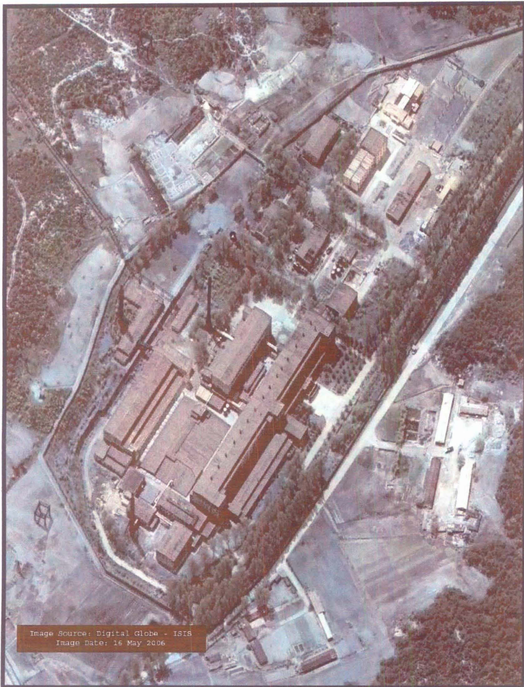
Radiochemical Laboratory at Yongbyon. Note the demolished corner near the bottom of the image in a facility whose purpose is unknown. The “canyon” where reprocessing occurs is a long, multistory building on the right
