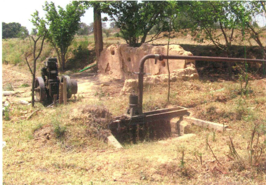
Uplift in groundwater table gave a spurt to tubewells due to which water table subsided
