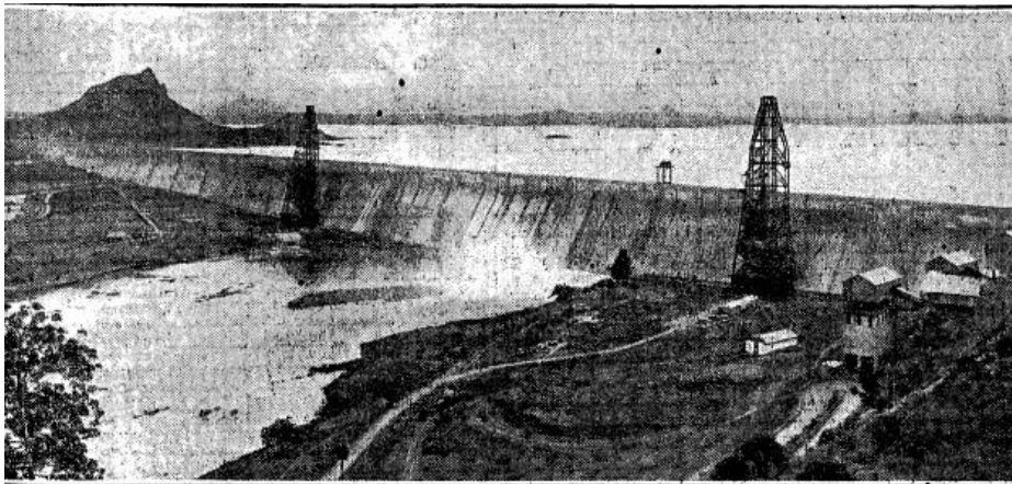
Figure 5: Mettur Dam: Overview of construction site, Times of India , August 1934.
