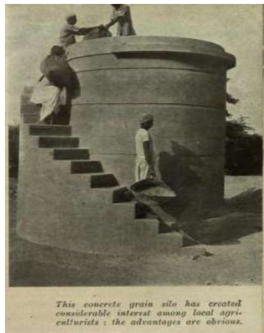
Figure 7: A Concrete Grain Silo: Rural India and Cement, Marg: A Magazine of Architecture and Art , Vol 1, No. 4 (1947): p.44
