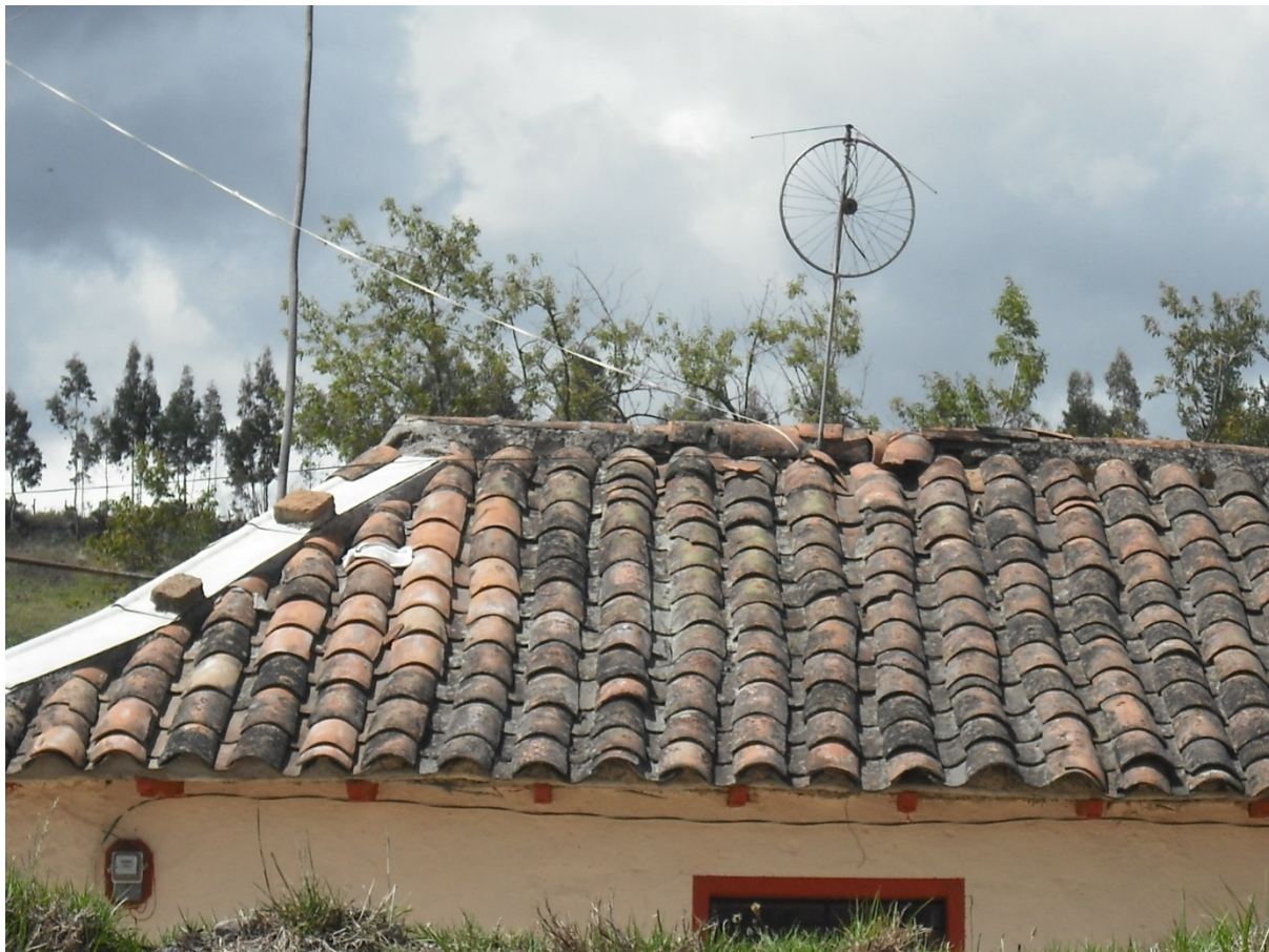
Figure 3 - Bicycle rim used as an antenna for signal reception
