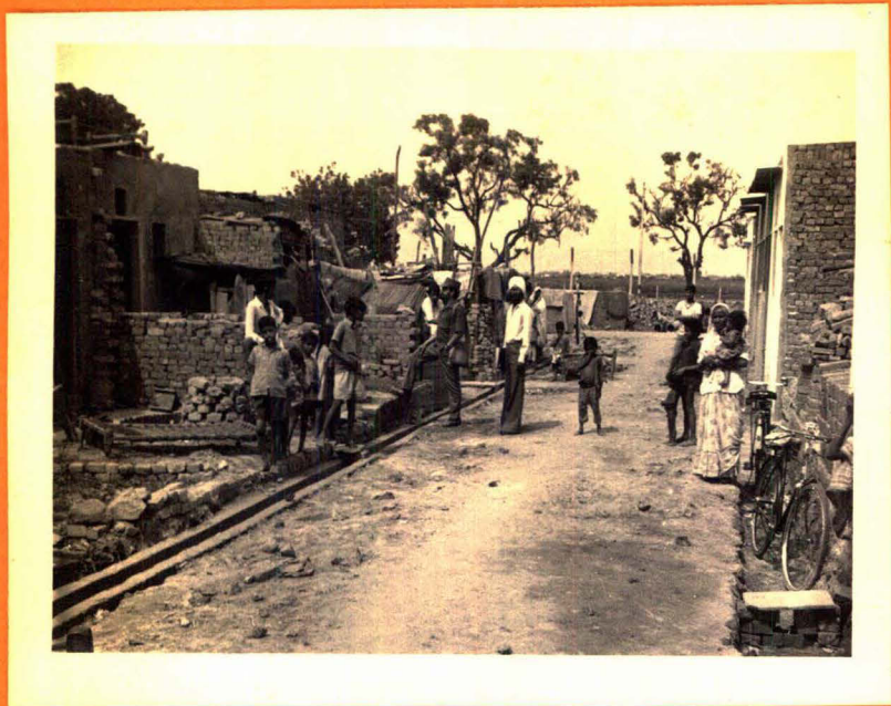
A VIEW OF STREET IN KHANPUR.
