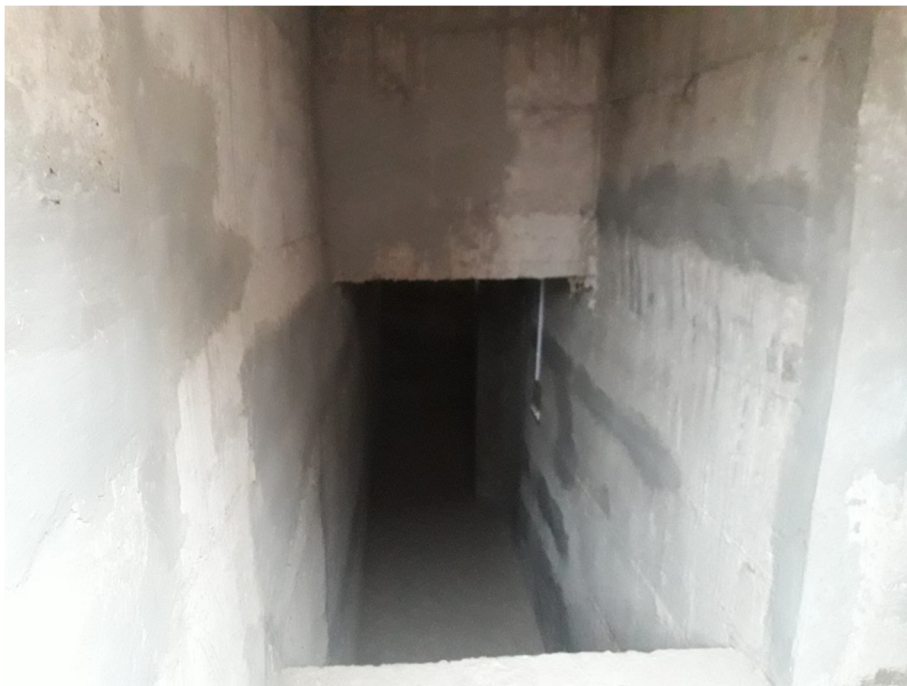
Community bunkers constructed in the village Rajpura (Photograph by Author)
