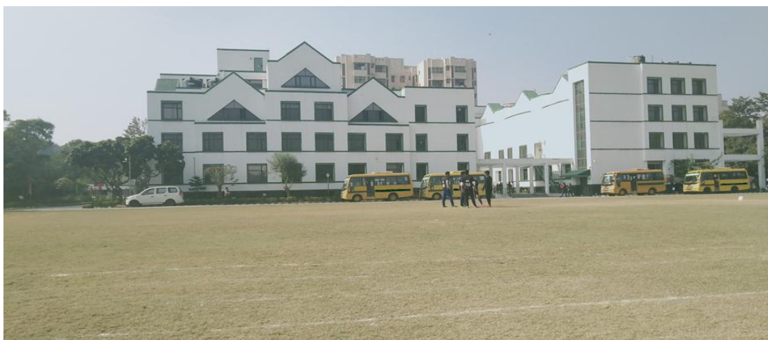
Figure 3.3: A side view of the building of PIS from the football field
