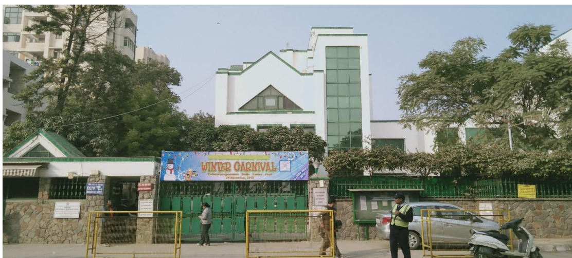
Figure 3.1: Main entrance of the school
