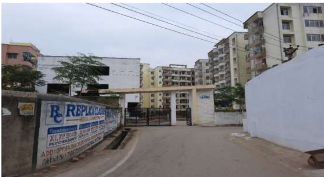
Plate 3.3 Apartment is constructed during 2018-19 in Jai Prakash Nagar locality
