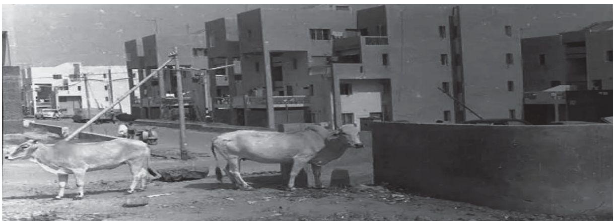
Figure 5: Newly constructed DDA flats Munirka, a 1976 photograph (Source: Seth, 2016).
