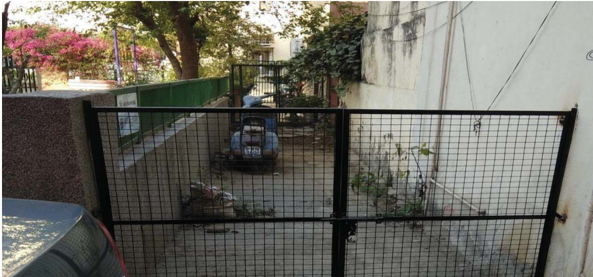
Figure 39: Earlier open, but now enclosed- a space turned into parking for two-wheelers at DDA flats Munirka. Picture clicked in spring 2018.
