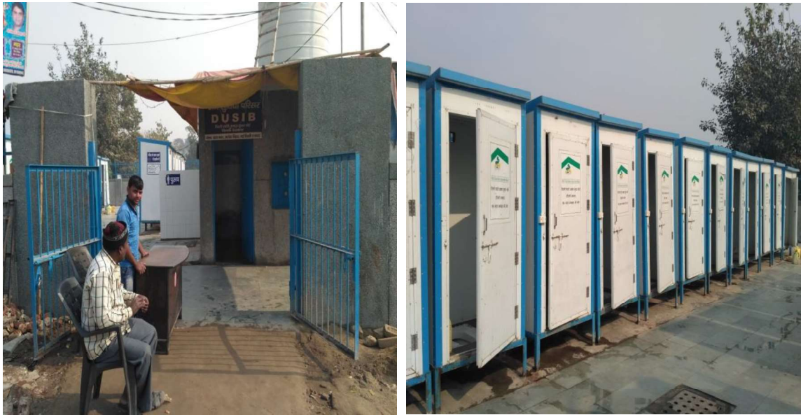
Figure 5.7: Newly constructed pay-per-use fabricated structured toilet blocks in Jailorwala Bagh slum, Azadpur. Photo captured by the Researcher.
