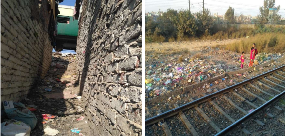
Figure 5.4: Railways tracks are right behind the wall of the houses. People have to cross the railways tracks to defecate in open in Seelampur, this rail route connects busy route of Old Delhi with Ghaziabad. Right hand side photo shows a child returning from defecation with green water bottle ( lota ) accompanied by a senior female. Photo captured by the Researcher.
