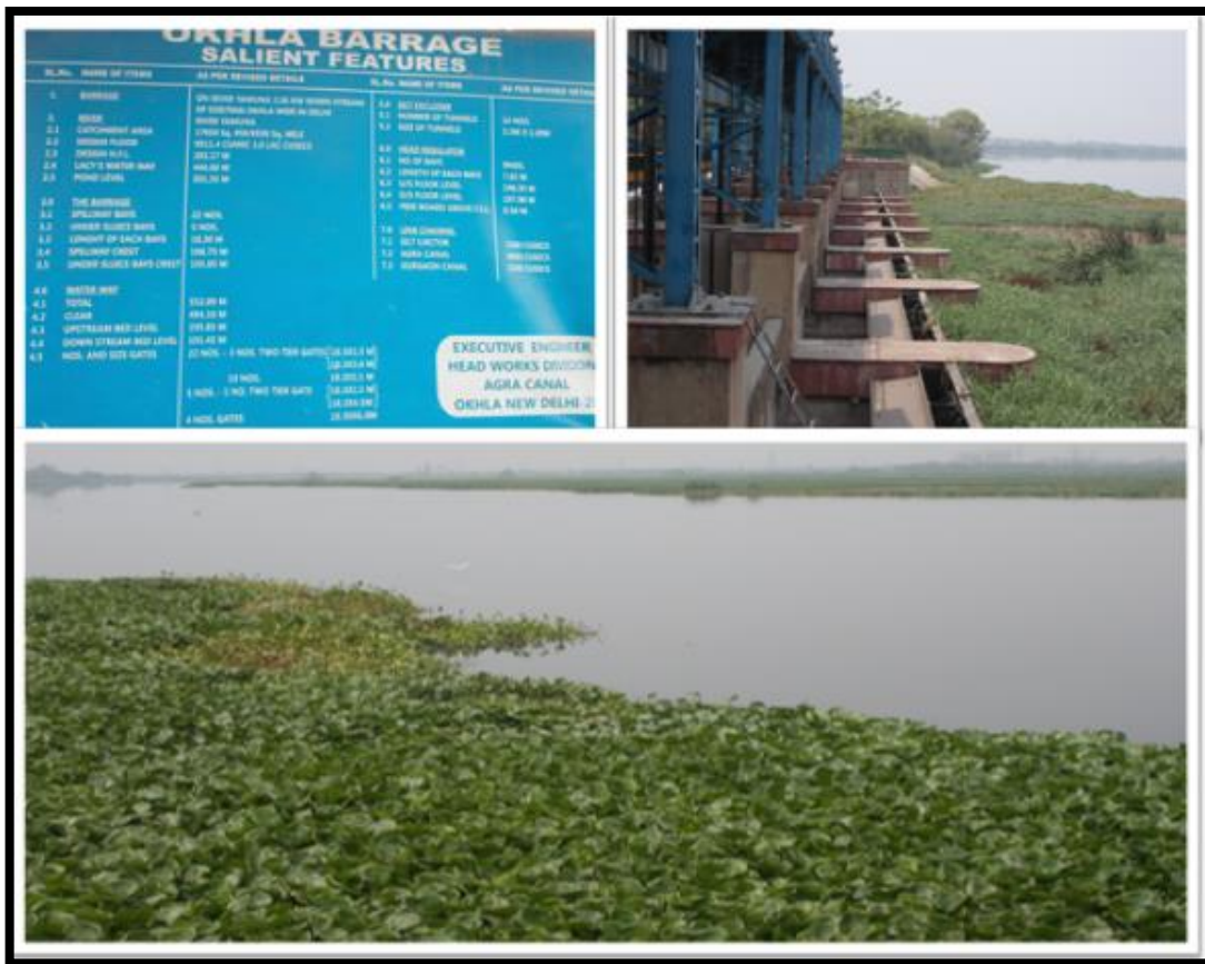
Source : Field visit to Okhla Barrage
