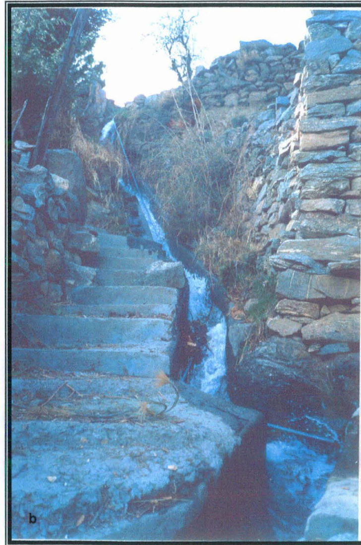
Plate V.1a & b Pucca Khuls diverting snow melt water to agricultural fields at Kalpa and Bre-Lingi villages respectively.
