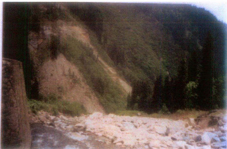
Plate 16: The man-made structure such as the one in the left foreground have increased the sites with potential slope failures.
