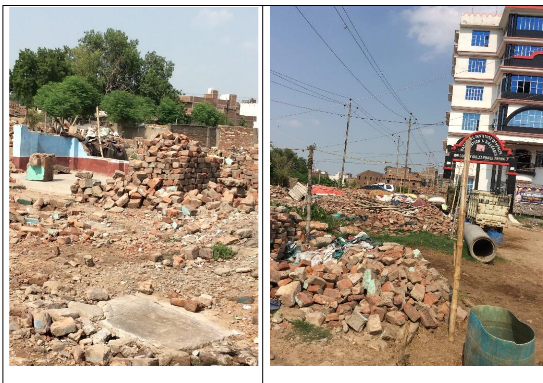
Image 7.1: Demolished slum and untouched multi-storey building
