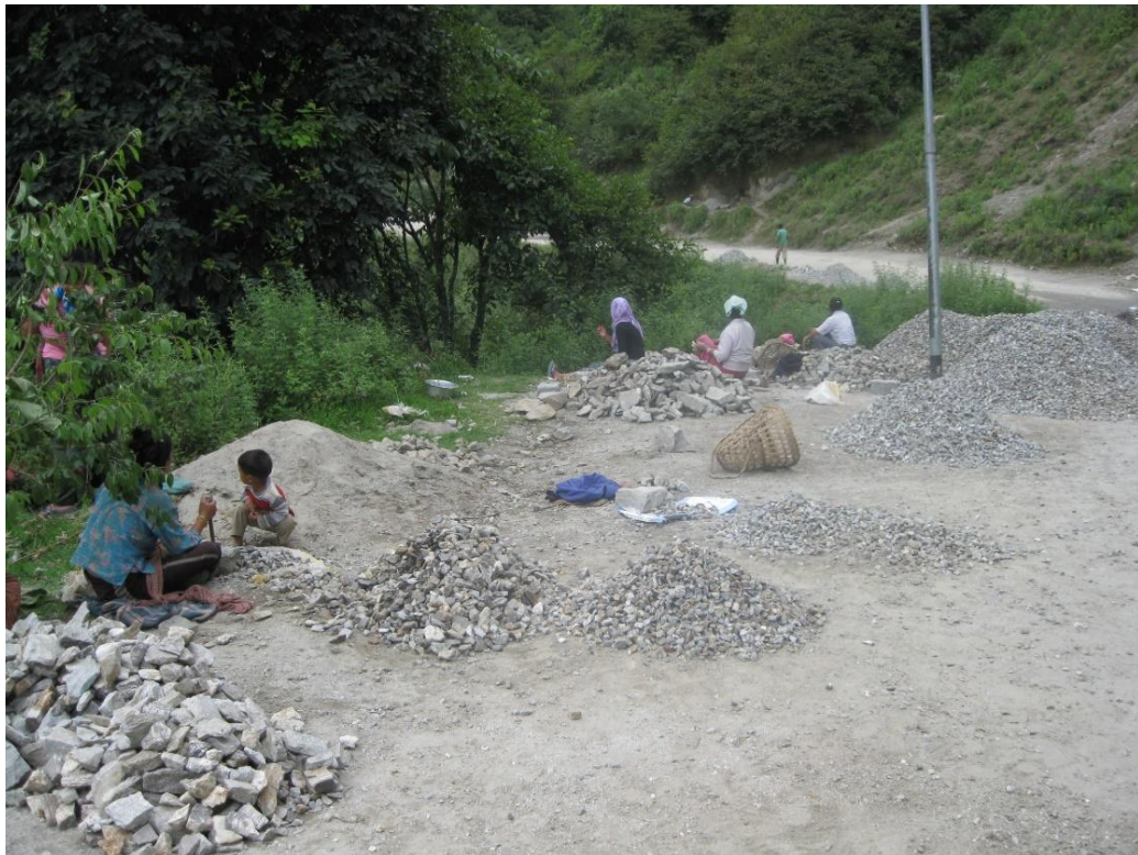
Figure 26: A road construction sight of India-China border region
