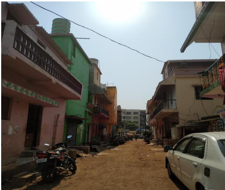
Plate 6.3 Multistoreyed constructions in the Sikharchandi basti
