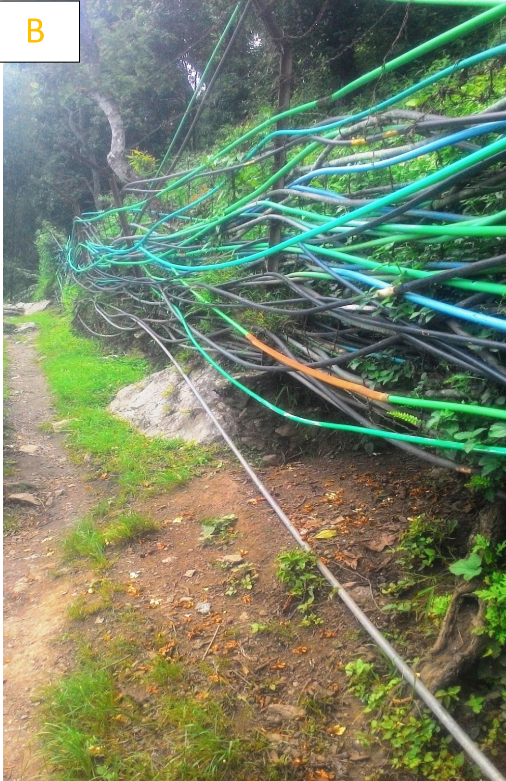
Source: Primary Survey, June 2017
