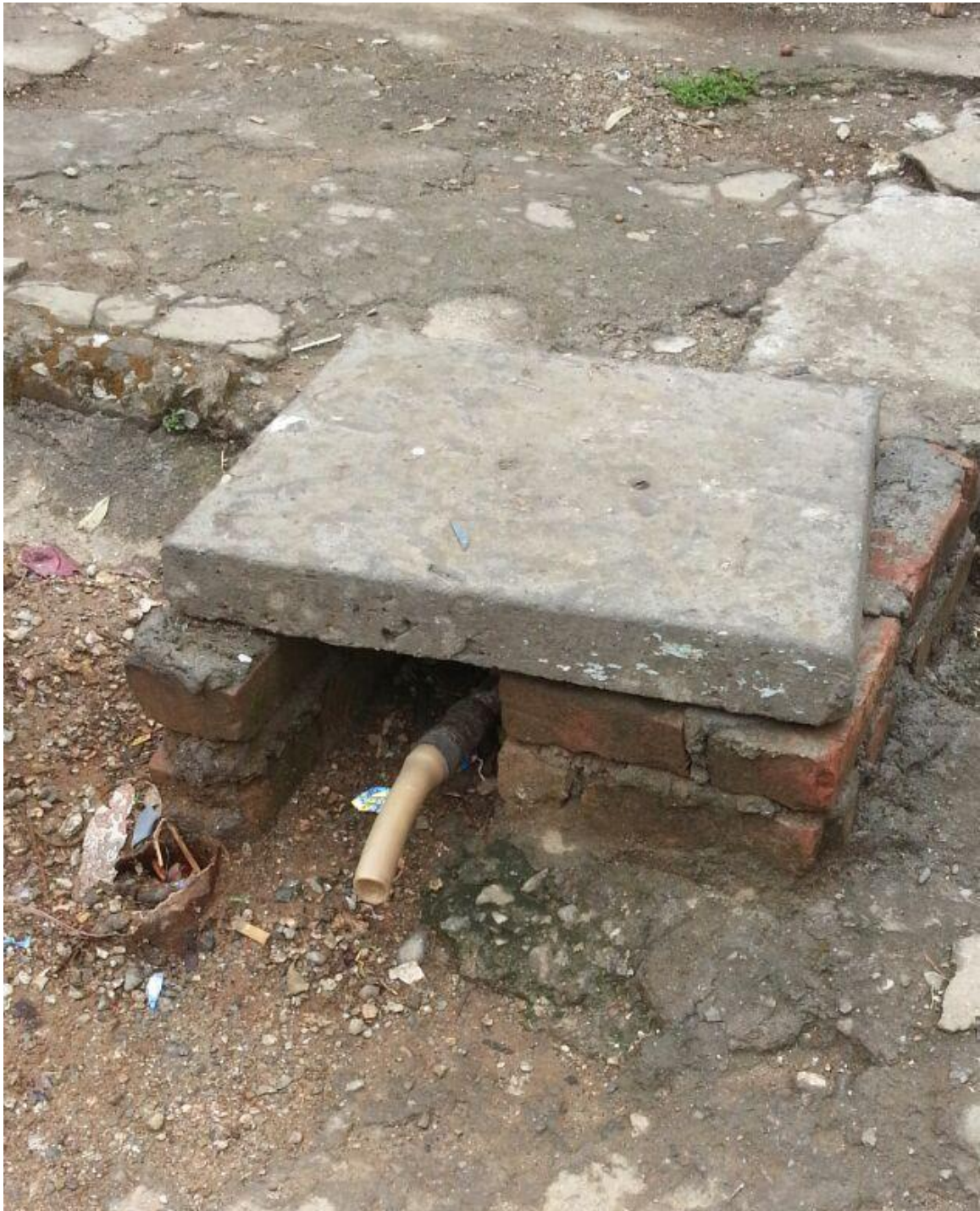
Image 1 The borehole located near hat bazaar Kalimpong which was closed down by the said political party
