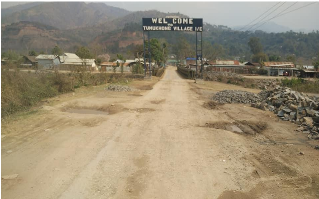
Tumukhong is a small village, an immediate downstream village within a kilometre of the Thoubal Multipurpose Project
