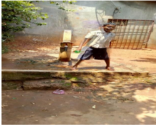
Plate 3: Unused public Hand pump due to heavy iron water (Bhimpur Area, Site 2) Plate 4: The condition of Public hand pump (Bhimpur Area, Site 2)
