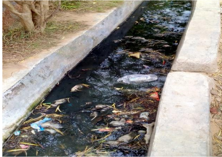
Plate 13: Drainage Condition (Naharakanta, Site-2)
