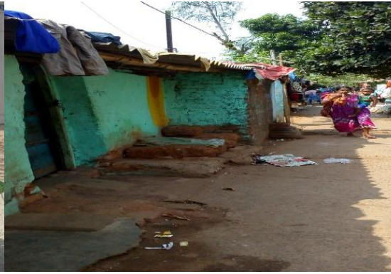
Plate 33: Houses condition of Sanitation workers
