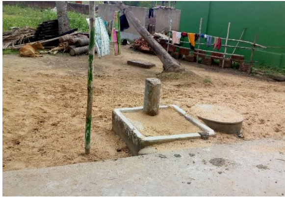
Plate 5: Malfunction of a Public Stand post in Naharakanta Site 2
