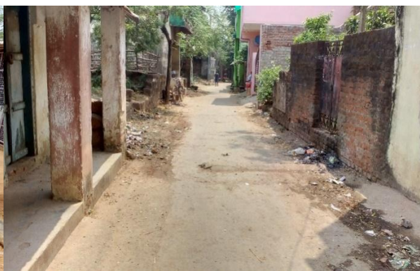
Plate 29: Poor Road Condition in Naharakanta Area, Site 2
