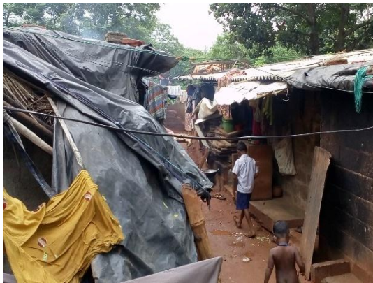
Plate 34: Poor Housing and Infrastructure condition of Sanitation
