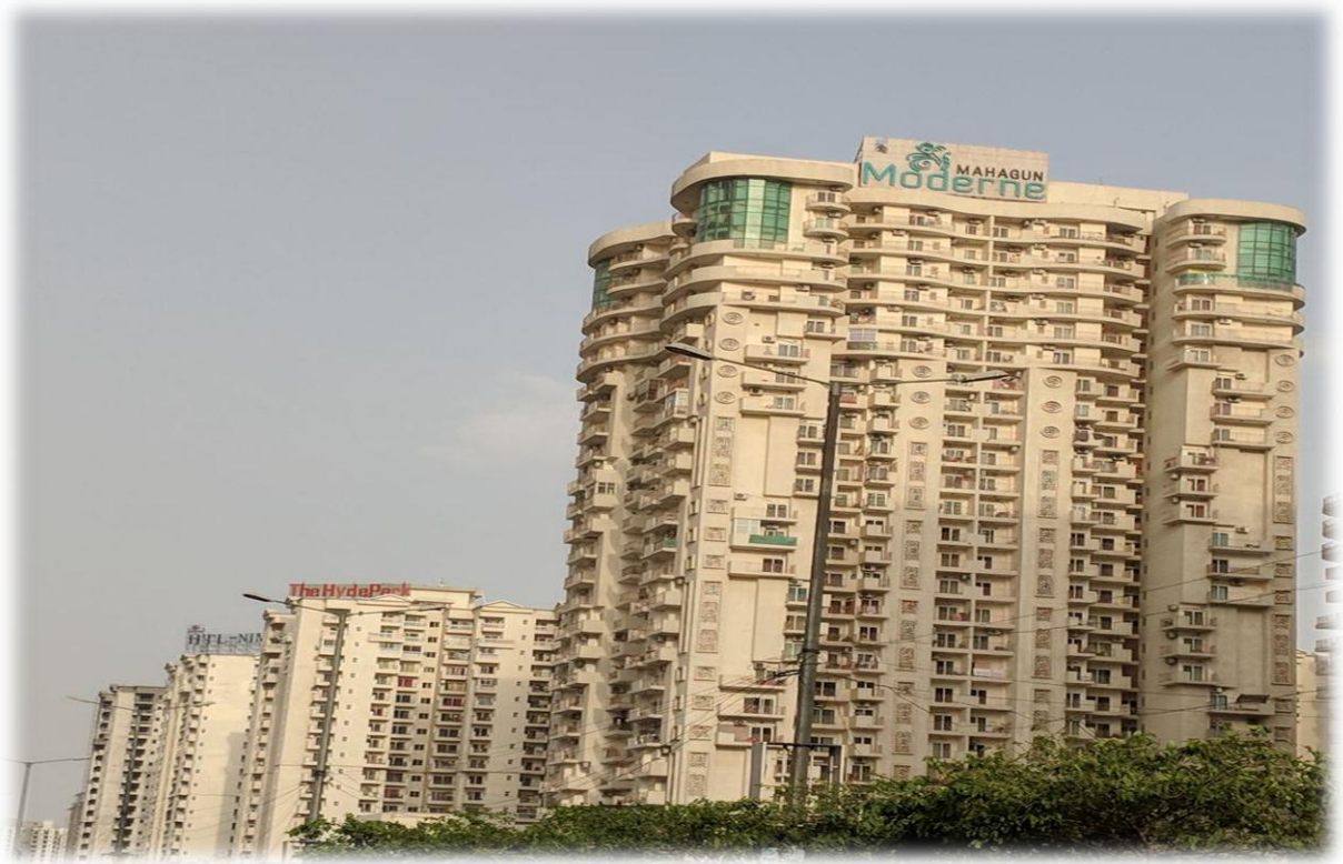
Figure 2: Residential Apartments in NOIDA.
