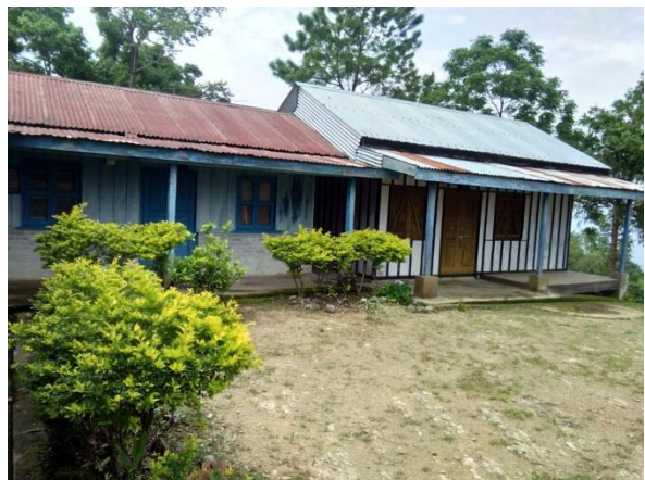
Tin roof with wooden cum brick wall house at Nzauna
