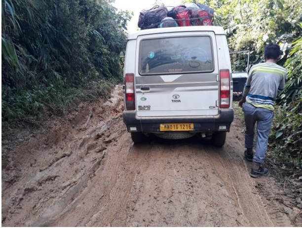
Condition of road towards Magulong
