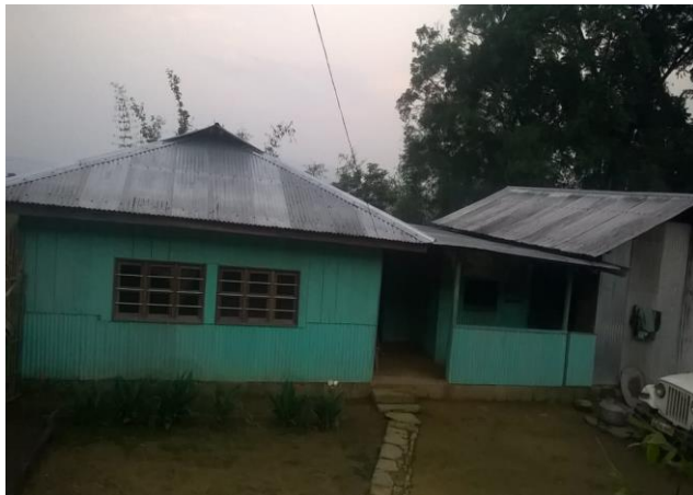
Tin roof with Tin wall house at Magulong
