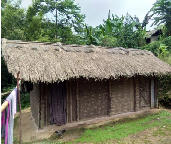
Traditional Thatched Roof with Bamboo wall house at Nzauna
