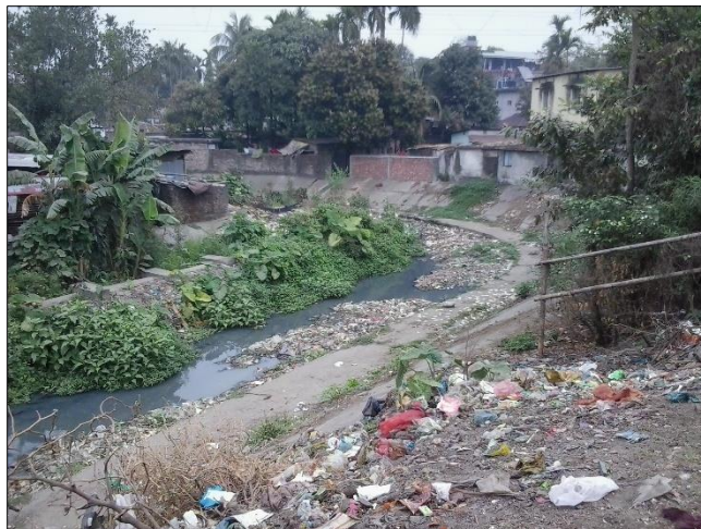
Plate-4.4: Choking of High Drains due to Solid Waste
