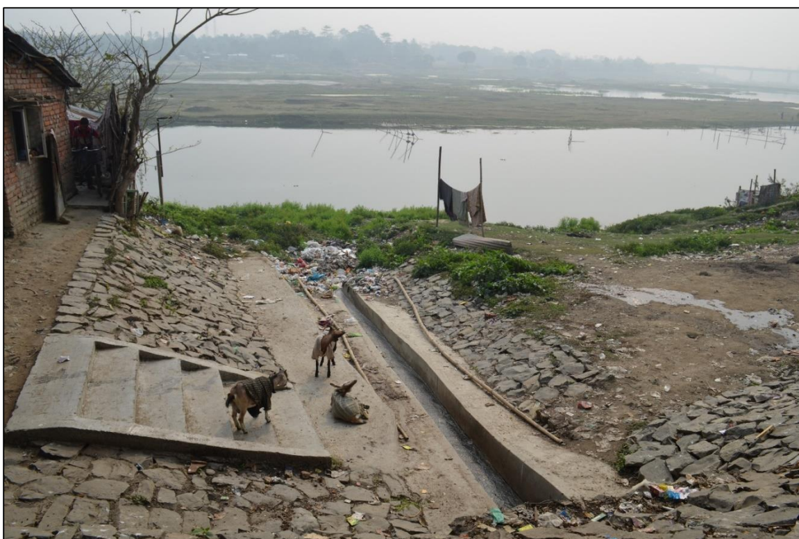
Plate-5.5: Cemented Main Drain, collecting household wastewater, is debouching into Mahananda River, English Bazar Municipality
