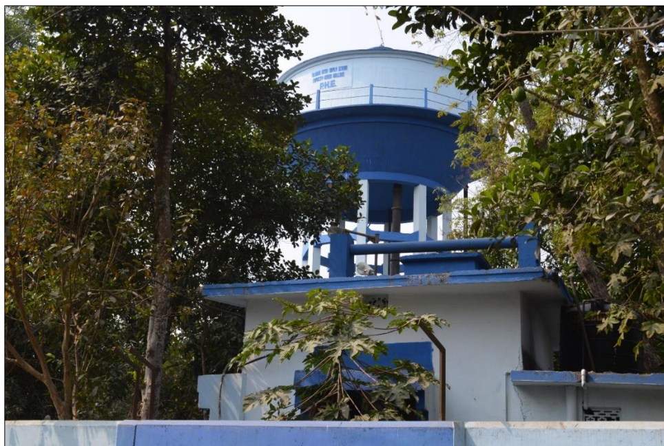
Plate-4.12. Overhead Reservoir used for storing water, with an attached pump house – operated and maintained by PHED, Haldibari
