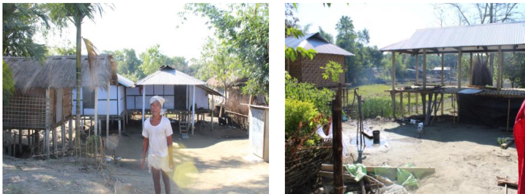
Grammar of Structures 57 : (L) An affluent homestead with a pig stay below. (R) House 'chang' under construction, replacing hay roof with tin and an elevated hand pump.
