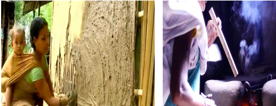
Products of a Resilient Grass: (L) A Bamboo house being plastered by mud. The practice is called Lepa. (R) A bamboo pipe called Chunga, used to build a blow air into the fire-place directly.
