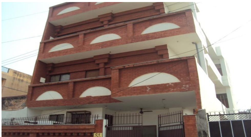
Figure 5.5: Anveshika New Building
