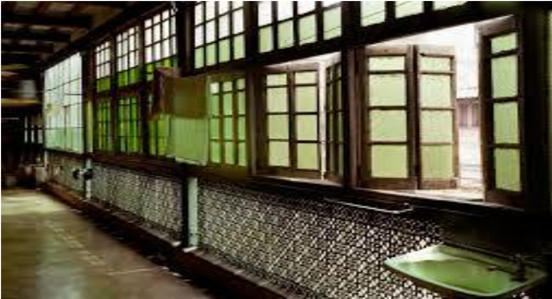
Figure 1: A typical North Kolkata gentry house, with wooden window structures called khori-khori in Bengali, and the ceiling also has wooden frames known as kori-borga in Bengali.
