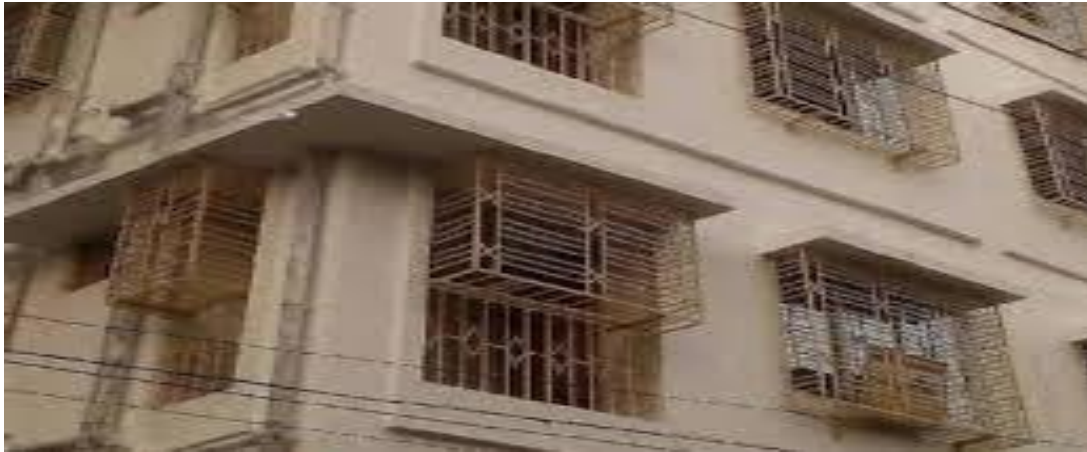
Figure 3: South Kolkata house built into an apartment at Jadavpur.
