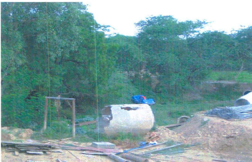
Bridge Construction over Water Body near Vasant Kunj, opposite to ICGEB
